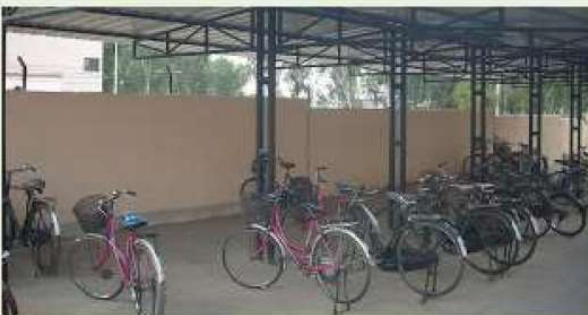
Shed Parking for Bicycles
